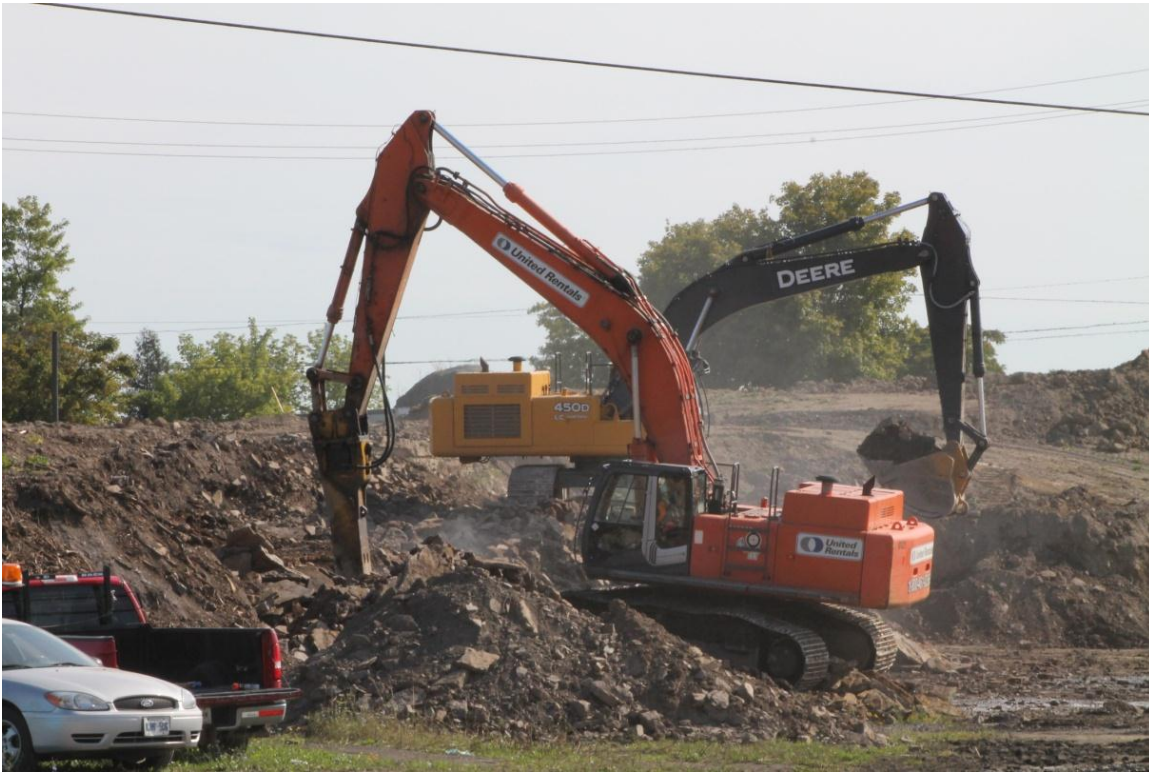
Photograph 1. Breaking and Removing Bedrock within Forebay and Detention Pond Footprint ↑
