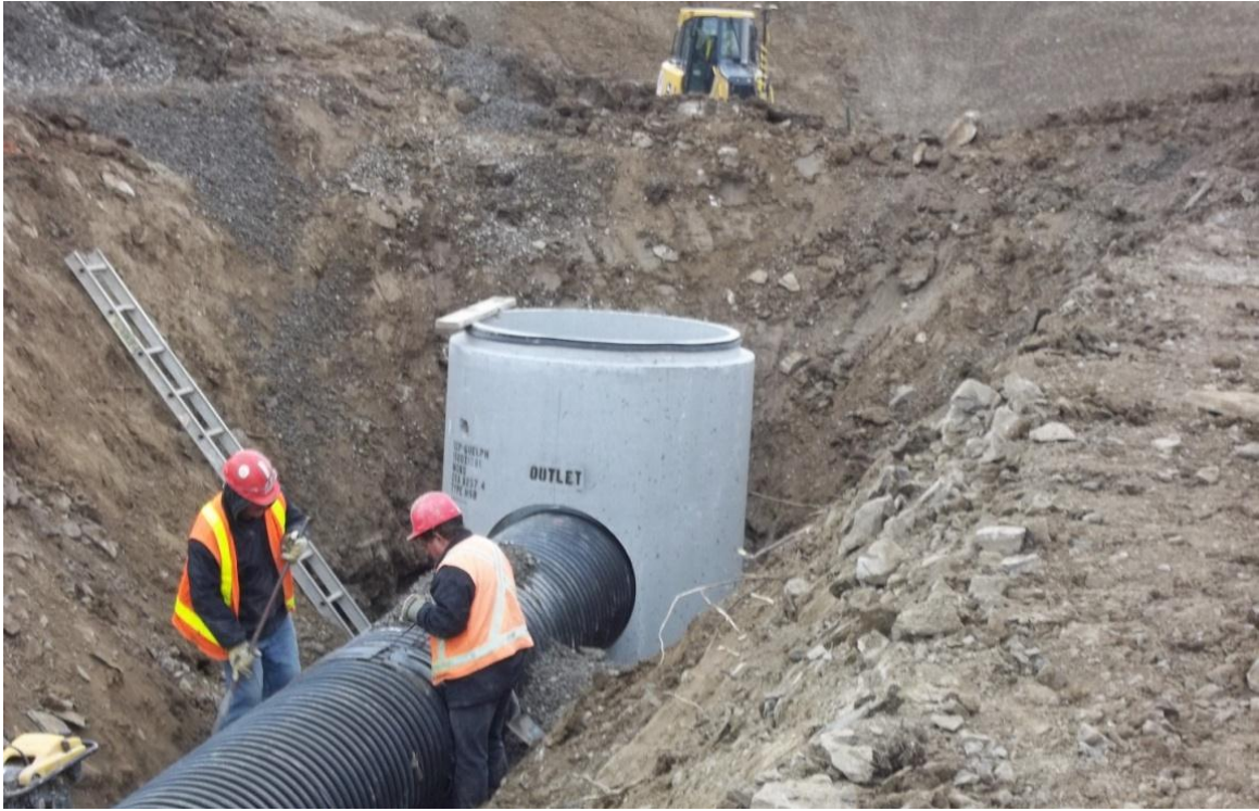
Photograph 7. Installation of Maintenance Hole with Detention Pond ↑
