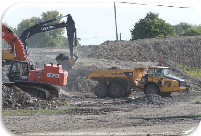
Braking and Hauling Rock from Forebay and Detention Pond Footprint
