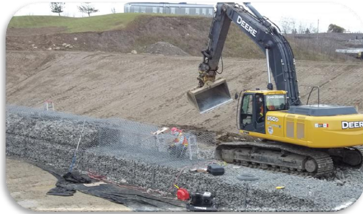
Construction of Gabion Walls within Detention Pond
