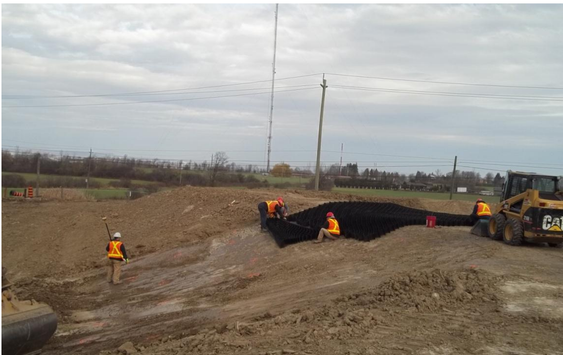
Photograph 4. Installation of Geoweb for the Overflow Weir ↑
