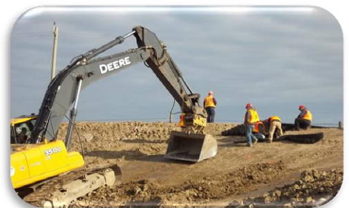
Deployment of Geoweb
