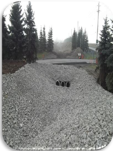
Perimeter Ditch with Culverts under the East Site Entrance Road
