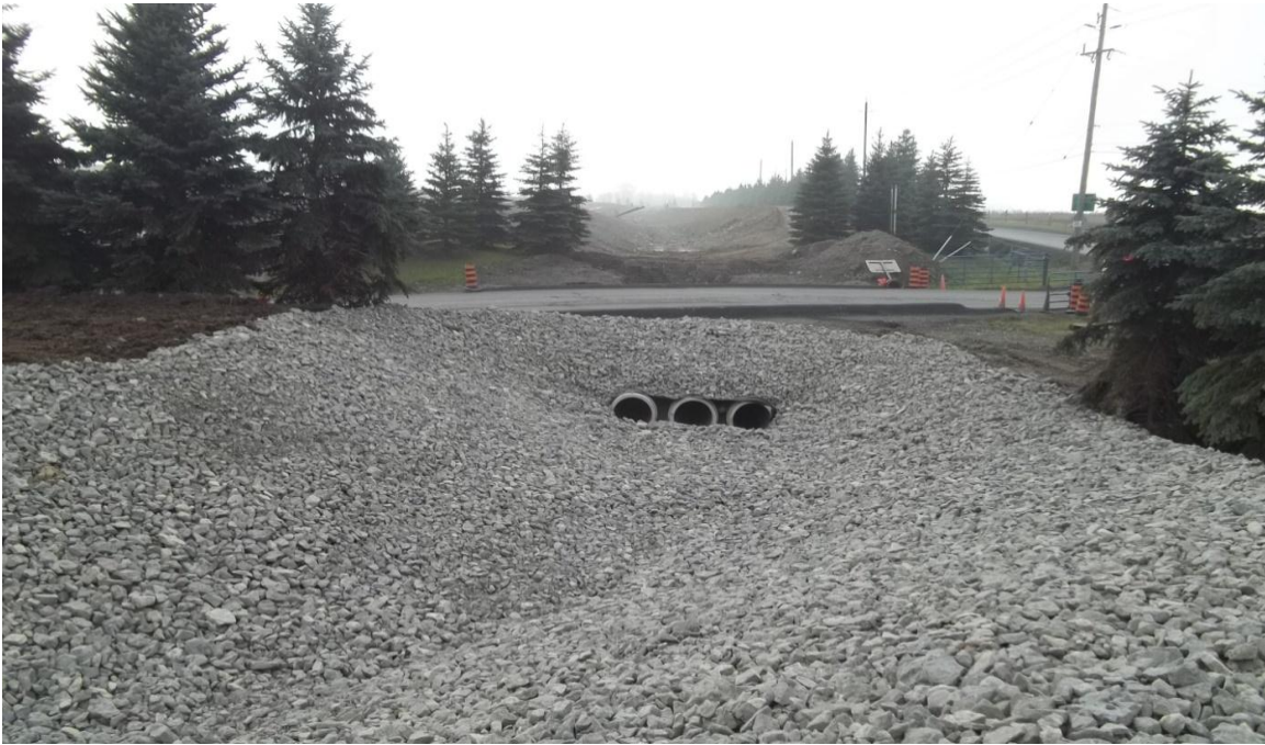
Photograph 9. Culverts under the West Site Entrance ↑
