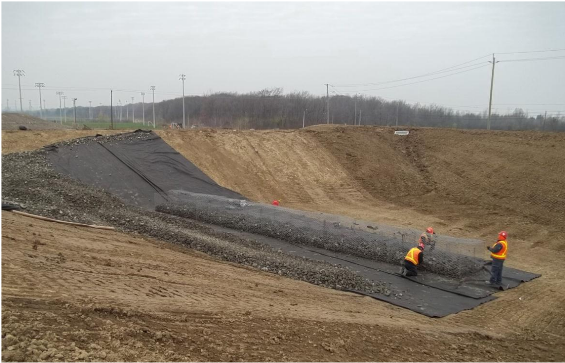
Photograph 3. Construction of Gabion Wall within Detention Pond ↑
