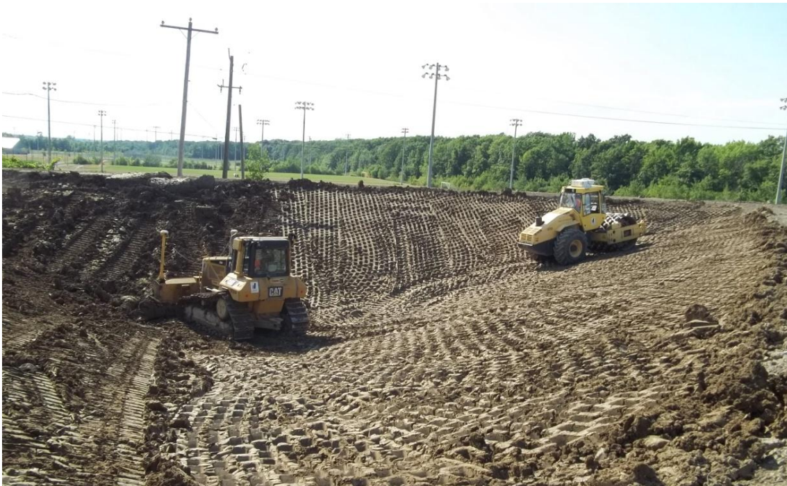
Photograph 2. Compacting Clay Liner within Forebay Pond ↑
