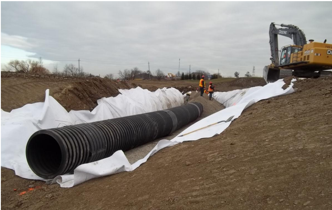
Photograph 6. Installation of Maintenance Hole at the Corner of Green Mountain Rd and First Rd ↑
