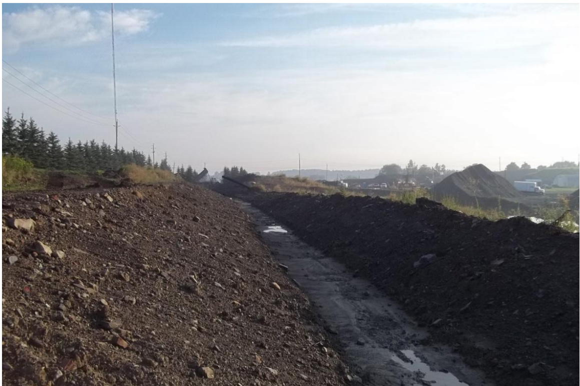
Photograph 8. Construction of Perimeter Drain Ditch ↑
