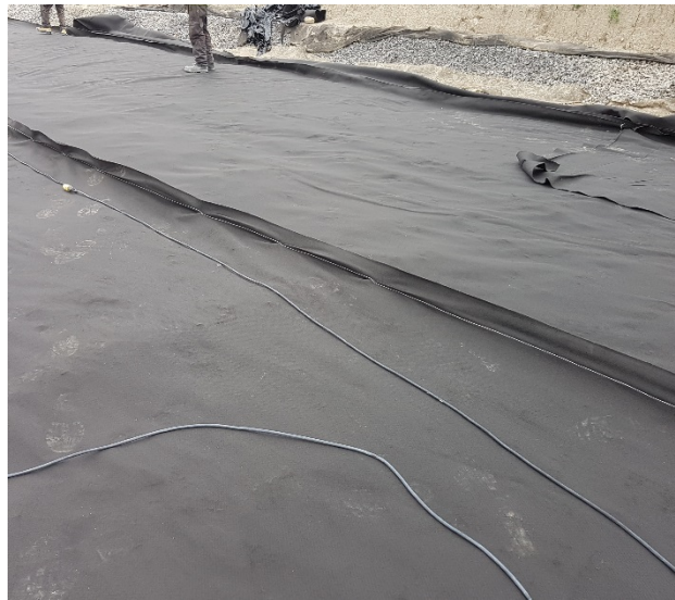
Photo 7 - Seaming of Geotextile
