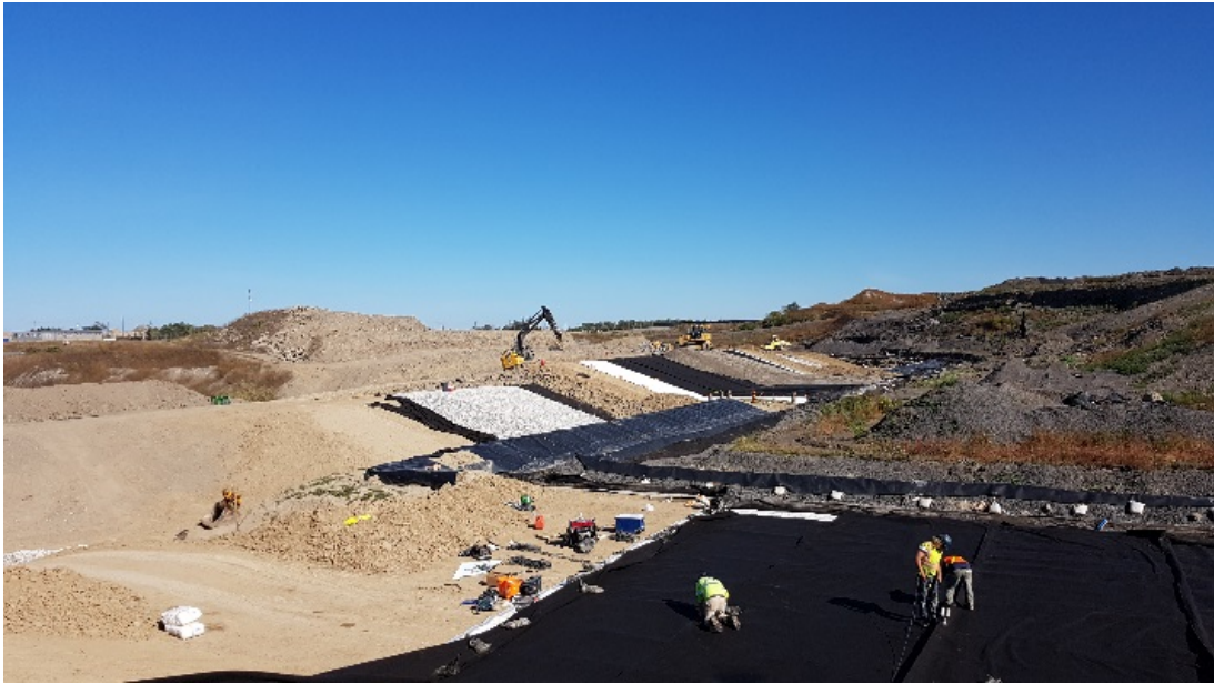
Photo 11 - Staged Construction of Base Liner Components
