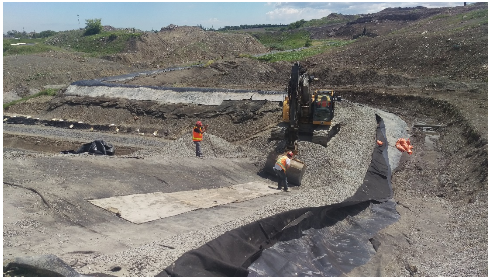
Photo 1 - Removal of the Existing Temporary Berm
