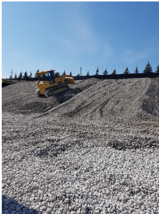
Photo 8 - Placement of Clear Stone for the Hydraulic Control Layer
