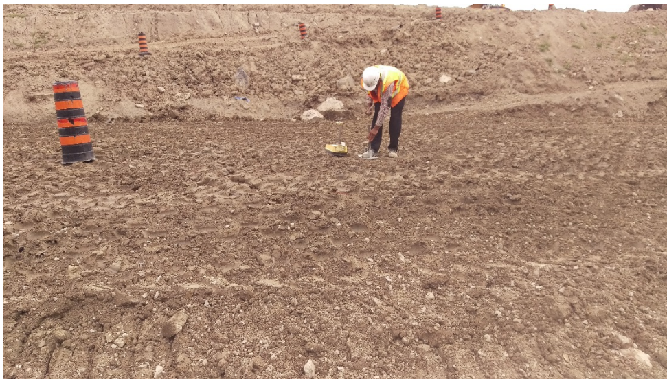
Photo 4 - Conducting In-Situ Compaction Testing of Clay Liner
