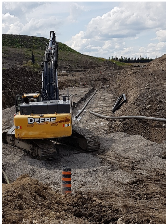
Photo 2 - Construction of Groundwater Collection Trench
