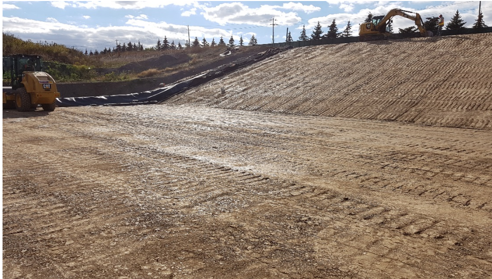
Photo 6 - Smooth Rolling the Final Lift of the Clay Liner
