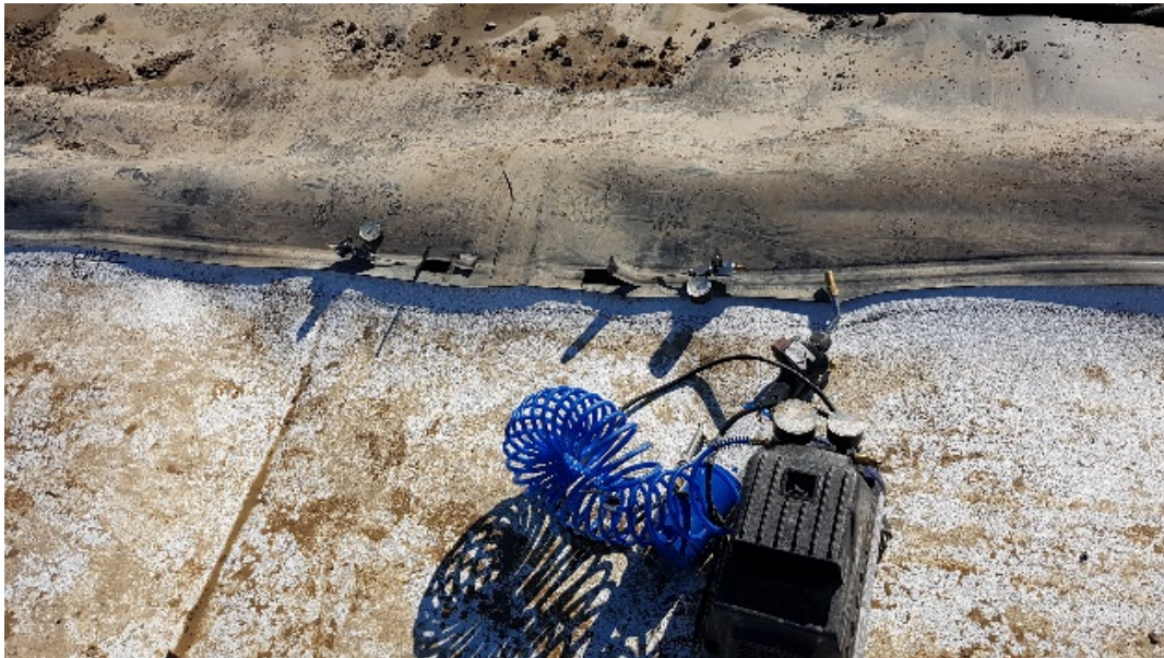
Photo 10 - Air Testing Welded Geomembrane Seam
