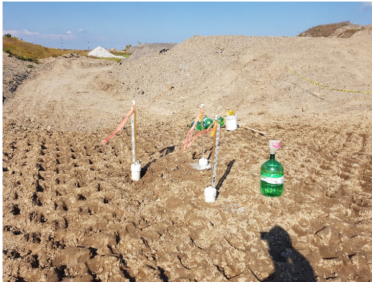
Photo 5 - Conducting In-Situ Hydraulic Conductivity Testing of Clay Liner
