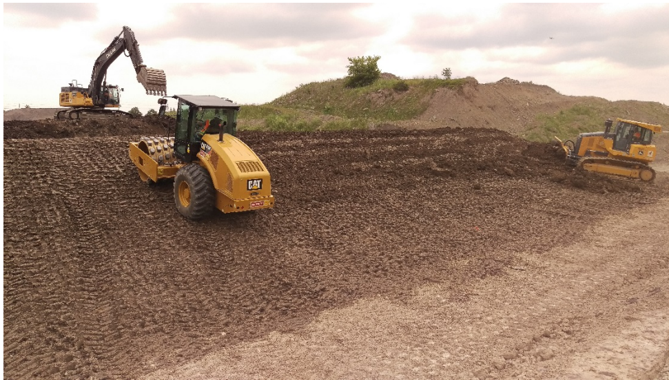
Photo 3 - Construction of the Engineered Fill Sidewall
