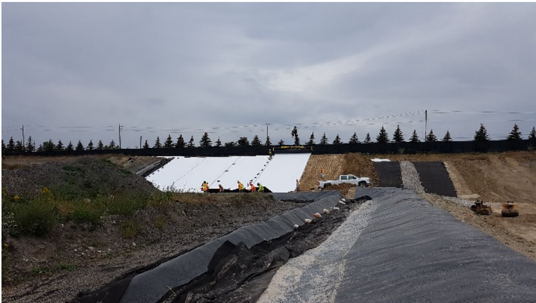
Photo 9 - Deploying Geomembrane on the Sidewall
