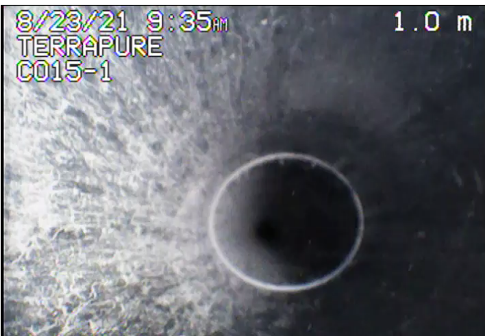
AMH - Access Point - Manhole @ 0.0 m. Starting Manhole: CO15-1
