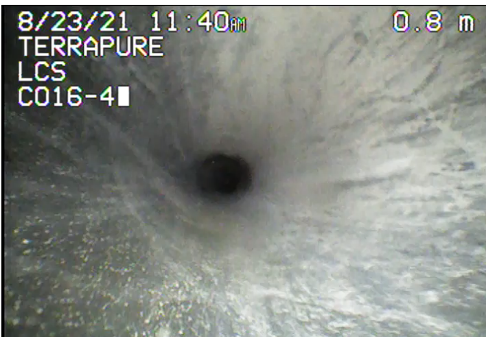
AMH - Access Point - Manhole @ 0.0 m. Starting Manhole: CO16-4
