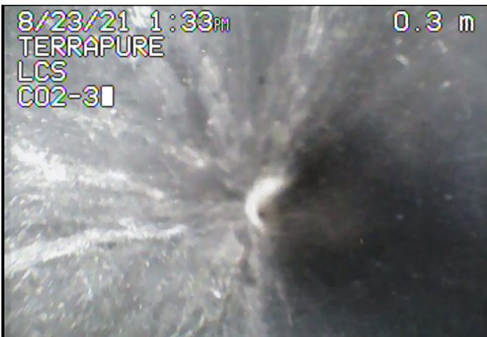
AMH - Access Point - Manhole @ 0.0 m. Starting Manhole: CO2-3
